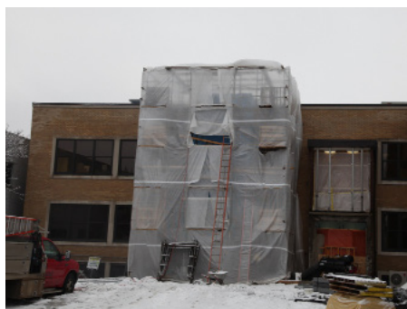
Building the elevator shaft.
