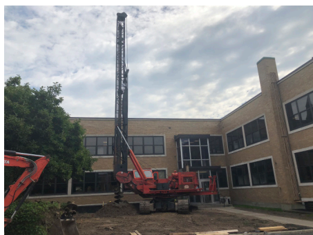
Breaking ground for the new elevator.
