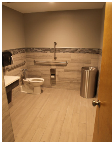
A renovated bathroom, more accessible for all of our clients.
