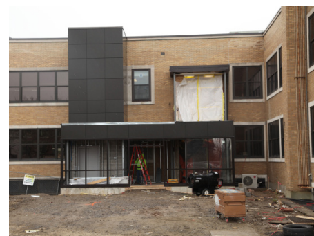
The elevator and new entryway.
